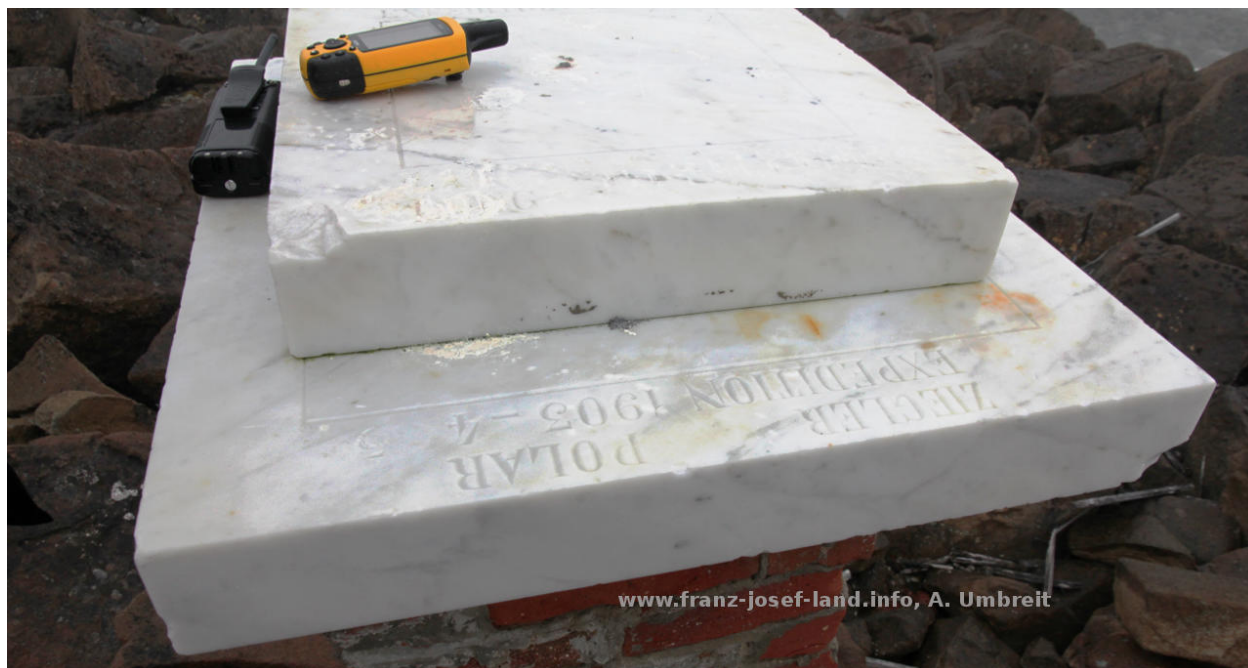
Fig. 8. The remains of Fiala's astronomical observatory at Teplitz Bay: the base that was constructed to hold the Repsold Circle loaned to the expedition by the University of Oslo (© Andreas Umbreit).
